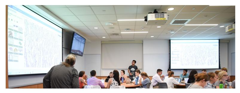
The new, larger classroom is set up with (10) 1920  $\times$  1200, 6,500-lumen NEC laser-hybrid projectors positioned on each of the four walls. The projectors and their accompanying ceiling-recessed screens are used to display the educational content.
